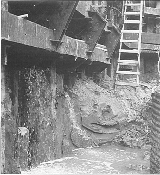
Plate 3 - A temporary excavation in marine mud in Junk Bay
