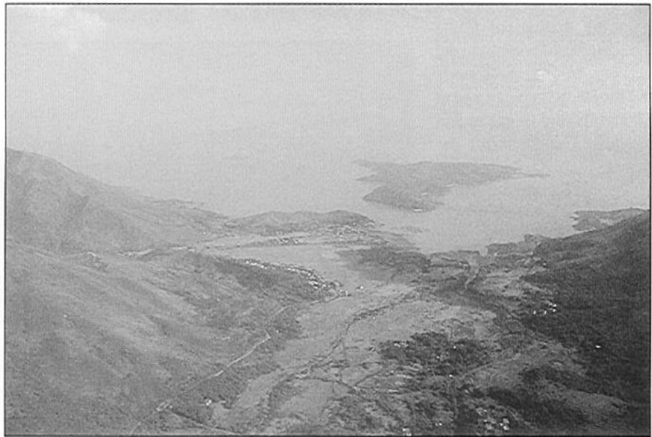
Plate 6 - Extensive marine geological investigations are in progress around Chep Lap Kok island, the site of Hong Kong's new airport
