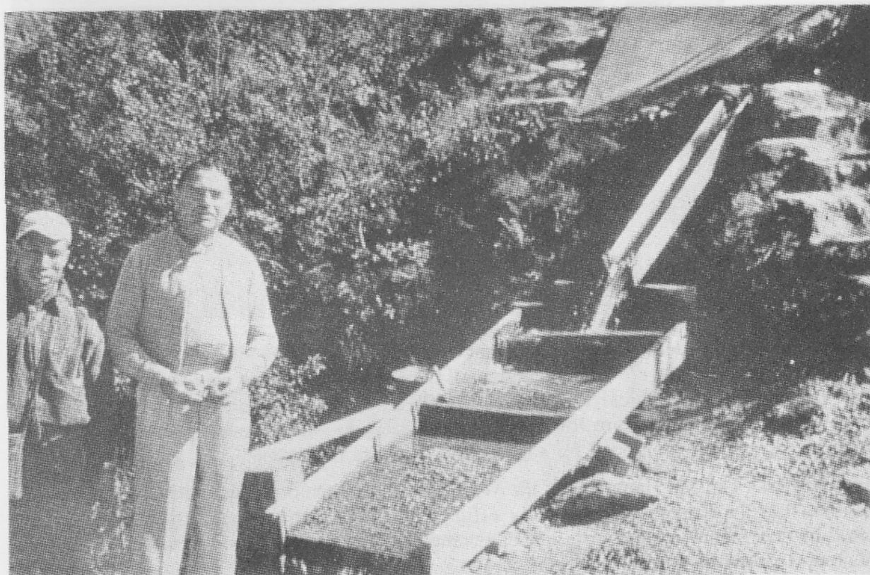
Plate 7 Sluice box used for separating galena in 1956. Professor S G Davis with sluice man
