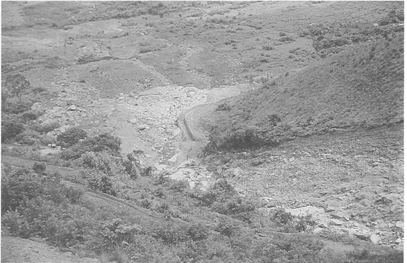
Plate 4 Constriction at the concrete stream intake, and the debris flow deposit spread out in Area 19 of Tuen Mun; note the small pond
